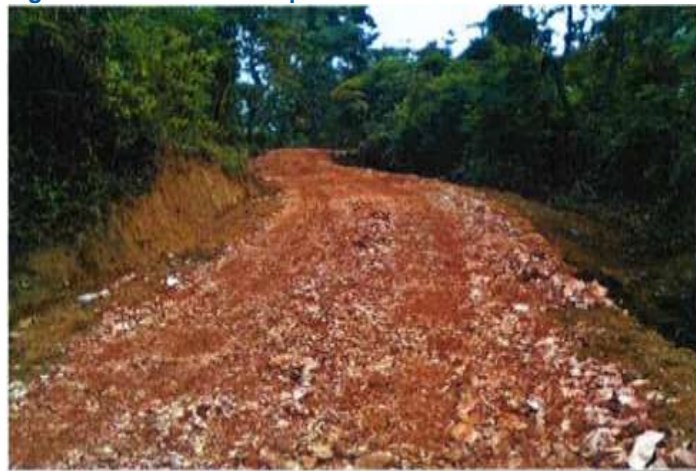
Figure 14: Low-cost compacted access road
