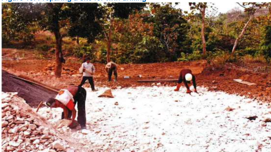
Figure 15: Preparing a site for twin drilling
